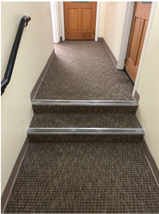
Engineering placed two step covers for owners to easily identify there is a step in this area. This should prevent people from missing the step and falling.
