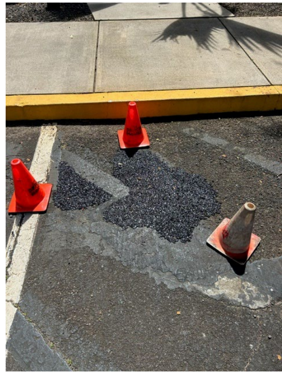
Engineering repaired a hole in the drive near the Coral ramp.
